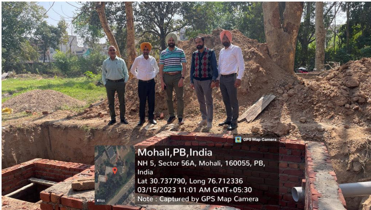
(Rainwater Harvesting System being constructed)
